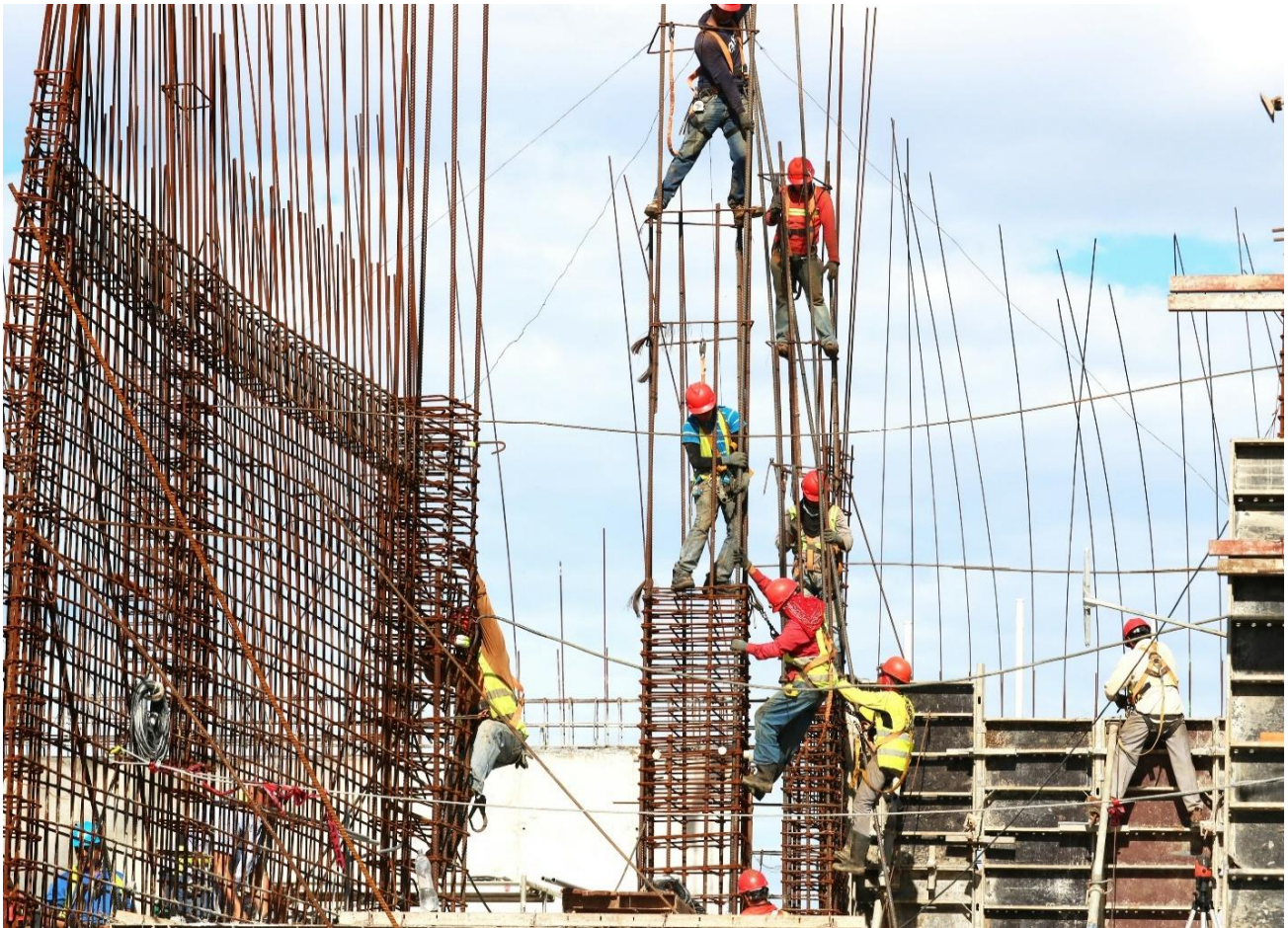
This image from Costa Rica demonstrates how the common construction process of building upward floor by floor means workers responsible for the preparation for concreting (rebar and form work) are always exposed to the sun. Photo by Josue Isai Ramos Figueroa, 2018. Unsplash . Public domain .
