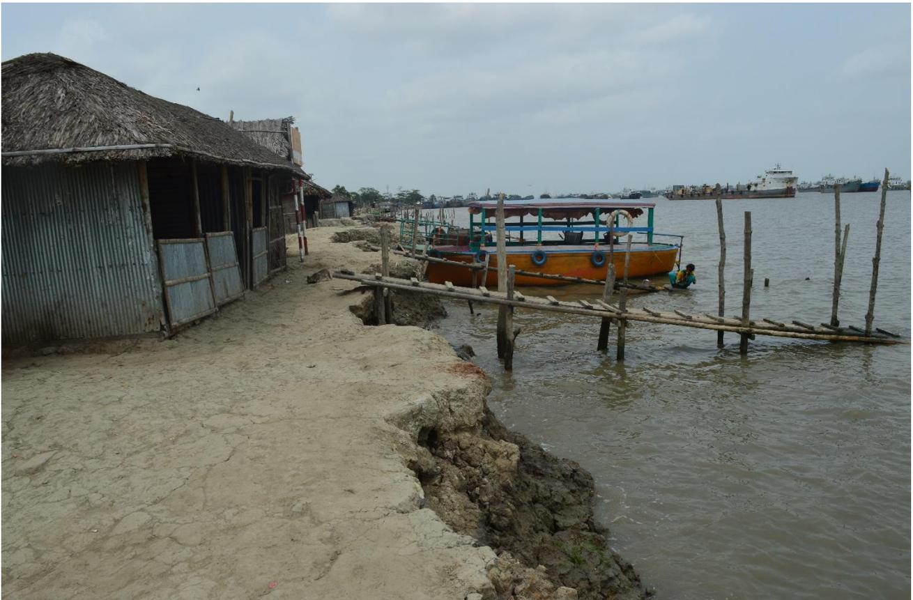
Fig. 7. The eroding embankment is slowly being "swallowed by the river." © Amrita Dasgupta. All rights reserved.
