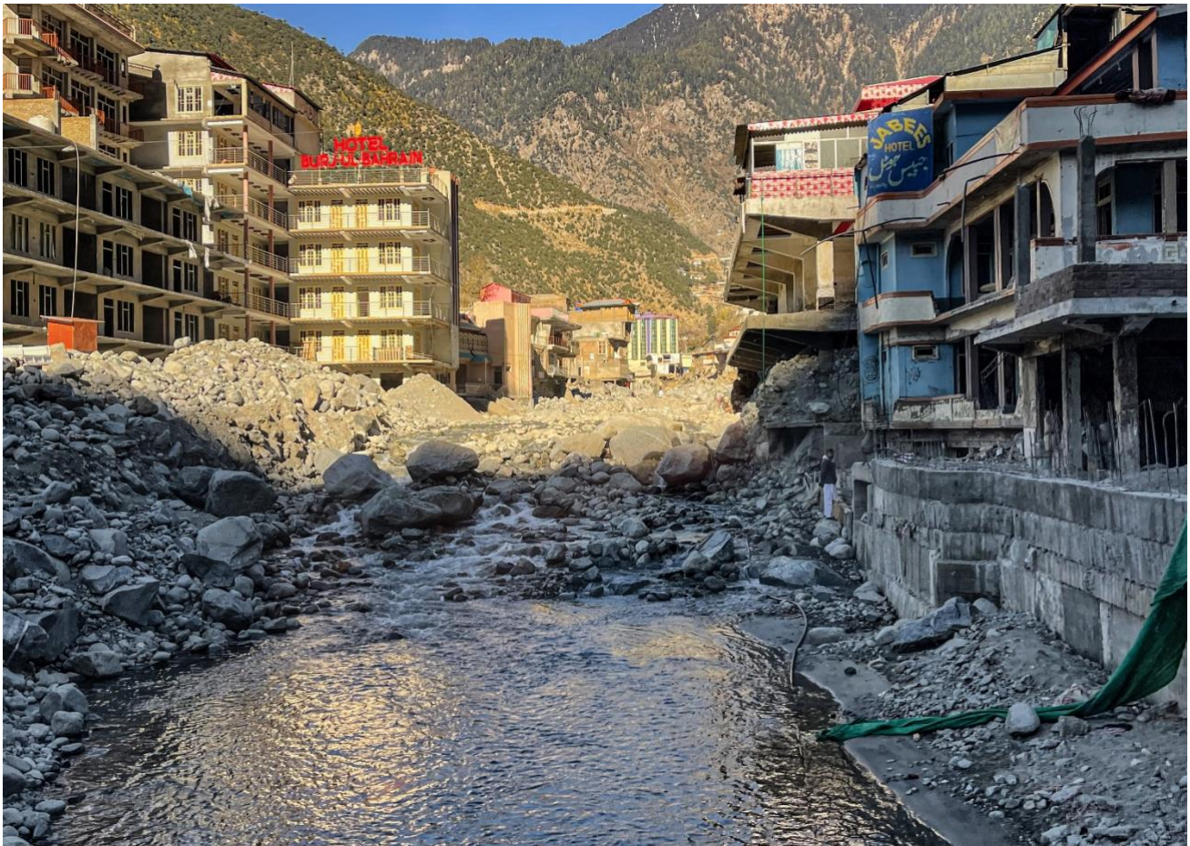
Fig. 2. Damaged road and buildings in Bahrain, Pakistan, October 2022, in the aftermath of severe flooding. © Anita Schneider on iStock. All rights reserved.
