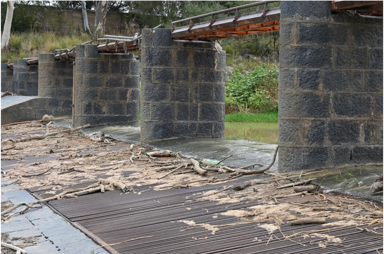
Traversa di Santa Domenica, Contrada Manganelli, Adrano, one of the main water-infrastructure features in the Simeto River. It was built in the 1960s to divert water from the river to the Contrasto hydropower plant, owned by ENEL Green Power. Since then, the environmental flow of the Simeto River has been compromised. Photo by Paolo Gruppuso. CC-BY NC 4.0 .
