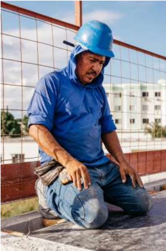
This worker rolling up his sleeves and with his helmet sitting too high on his head demonstrates what may be a trade-off between risks—immediate thermal comfort being privileged over longer-term risks of UV-protection and physical impacts/trauma. © 2023 JSB Co. on Unsplash. All rights reserved.
