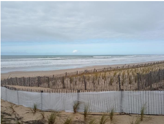
(Left) Human-made dunes: planting marram to trap the sand. Lacanau Ocean Beach, France. (Right) Hybrid dunes in Peniche, Portugal. Photos by Joana Gaspar de Freitas. CC BY 4.0 .
