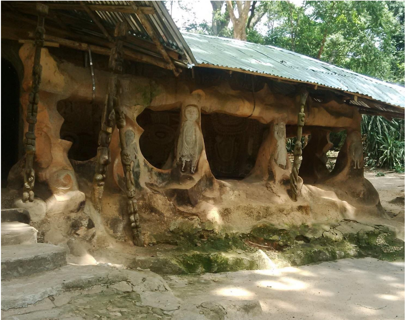
Fig. 6. Structural wooden caryatids at Osun Grove. Photo by Joseph A. Adedeji. CC BY-NC 4.0 .
