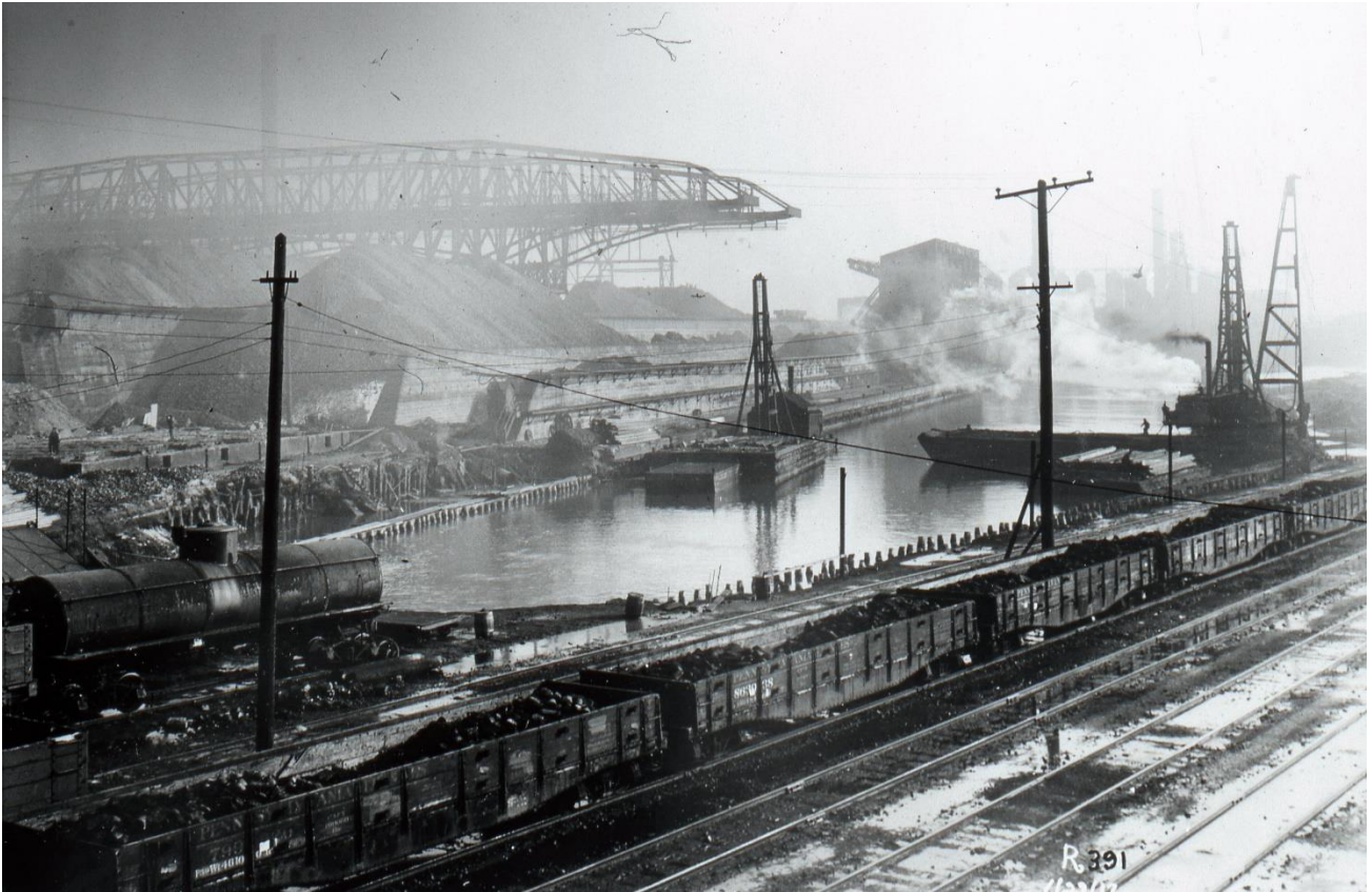
South Slip at South Works, 1917. This artificial inlet received ore and coal to be distributed by rail cars within the steel plants. Note the coal mountain within the ore walls just beneath the gantry cranes. Courtesy of the Southeast Chicago Historical Society [Archive ID: 1983-100-d22]. All rights reserved.
