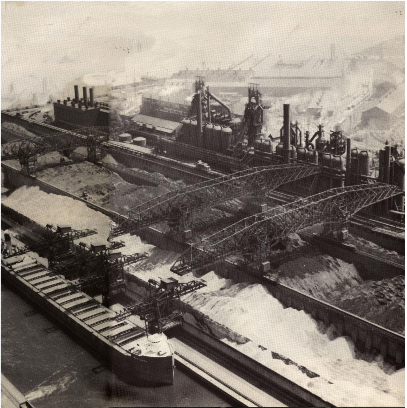
Fig. 7: Barges ready to unload cargo for storage with lime and ore between the ore walls. The buildings are a power station on the left and, in the center, behind the gantry cranes, what were the world's two biggest blast furnaces. South Works Anniversary Book: Steelmaster for 75 Years , [undated] ca. 1955. Courtesy of the Southeast Chicago Historical Society. All rights reserved.
