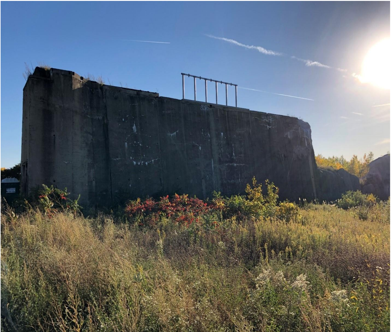
Fig. 8: Ore wall segment at South Works, October 2022. © John R. McNeill. All rights reserved.
